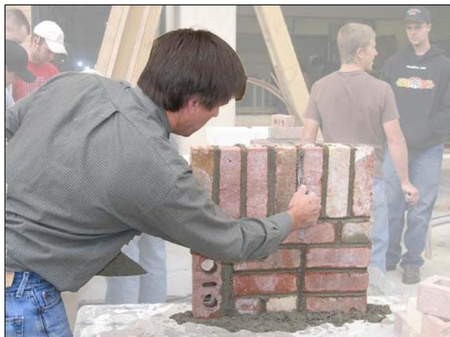
**Figure 10:** Mock masonry wall construction and brick laying familiarization.
