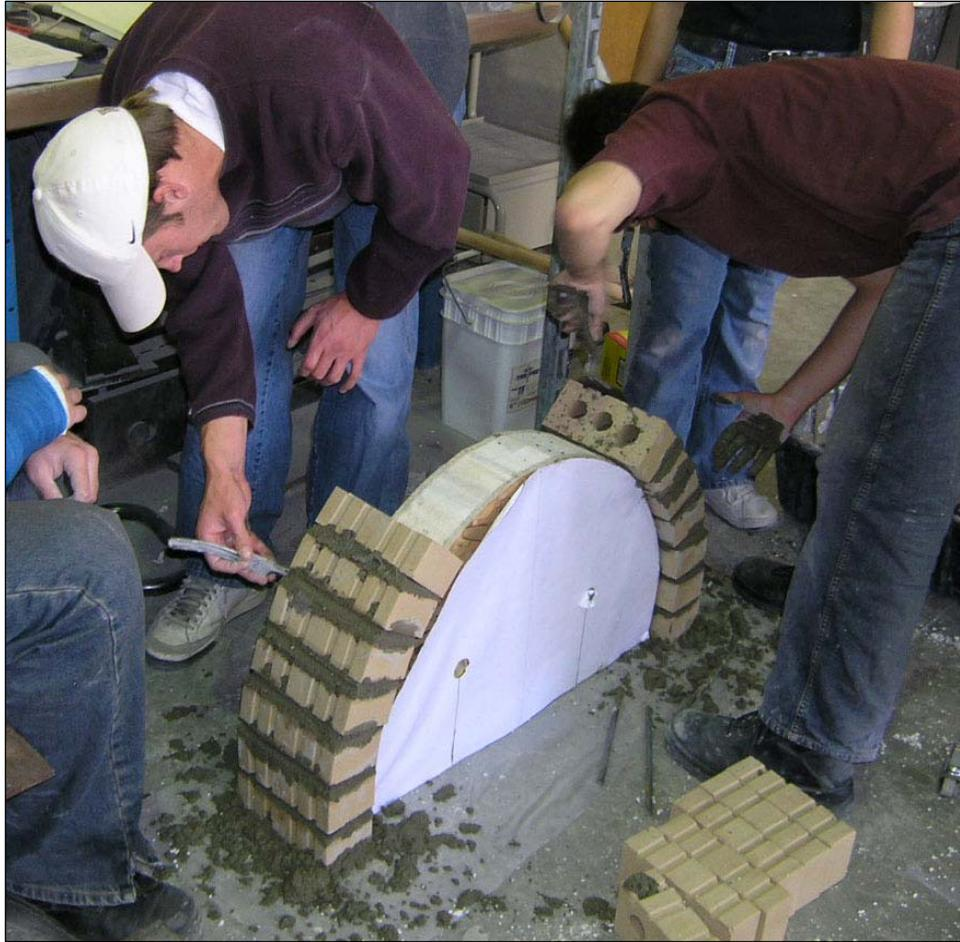
**Figure 11:** Masonry arch construction
